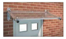
**4.7** Reposition canopy and secure with the recommended fixings (Fischer SXR 10x60mm).
