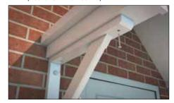
3.5 Secure the canopy to the brackets using the pre-drilled holes and recommended fixings. (Fischer Pozi ZP 5x50mm)
