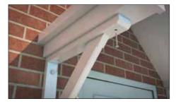
2.5 Secure the canopy to the brackets using the pre-drilled holes and recommended fixings. (Fischer Pozi ZP 5x50mm)
