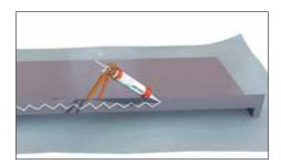
**8.5** Apply mastic sealant to the rear of the flashing upstand while on the ground. Use protective sheeting underneath the canopy.
