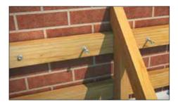
**6.4** Secure the canopy through the timber frame at a minimum of 300mm centres using the recommended fixings and plugs (Fischer SXR 10x100mm).
