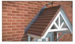
**2.6** When the canopy is fully secured a second mastic sealant can be applied.
