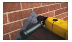
2.3 Fix canopy by drilling (drill bit size M10) through the flashing upstand at a minimum of 300mm centres.
