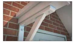
**5.4** Secure the canopy to the brackets using the pre-drilled holes and recommended fixings. (Fischer Pozi ZP 5x50mm)
