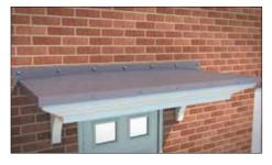
**7.6** When the canopy is fully secured a second mastic sealant can be applied.
