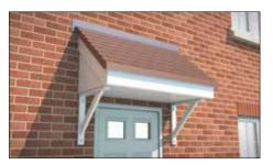
**5.2** Centre the canopy position, ensuring equal distance at either side, before pushing back to contact with the wall.
