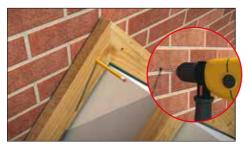
**3.3** With canopy in position, mark and drill positions for all fixings. Drill bit size M10.
