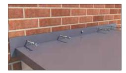
8.6 Secure the canopy by drilling through the flashing upstand at a minimum of 300mm centres. Use recommended fixings and plugs. Drill bit size M10. Continued >
