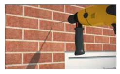
**4.3** Drill holes for first bracket. Drill bit size M10.
