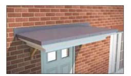
7.2 Centre the canopy position, ensuring equal distance at either side, before pushing back to contact with the wall.
