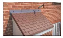
**5.5** When the canopy is fully secured a second mastic sealant can be applied.
