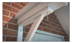
**6.5** Secure the canopy to the brackets using the pre-drilled holes and recommended fixings. (Fischer Pozi ZP 5x50mm)
