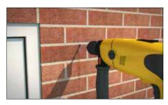
1.3 Fit brackets; mark positions and drill holes for first bracket. Drill bit size M10.
