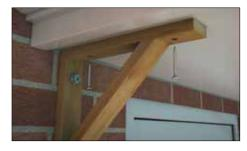
7.4 Secure the canopy to the brackets using the pre-drilled holes and recommended fixings. (Fischer Pozi ZP 5x50mm)
