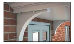
**7.5** Position the GRP Kneeler supplied and fix with polytop pins.
