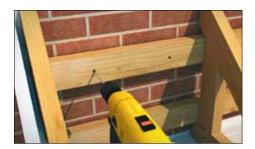
**6.3** With canopy in position, mark and drill positions for all fixings. Drill bit size M10.
