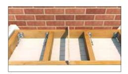
**8.3** Insert fixings. Do not fully tighten before levels have been checked and corrected.
