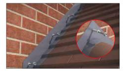
**2.4** Fix canopy using the recommended fixings and plugs (Fischer SXR 10x60mm).
