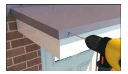
**8.7** Pre-drill holes using a M6 drill bit. Holes should be 50mm in from all corners and spaced at Max 500 ctrs.
