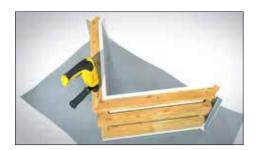
**3.1** Drill holes for fixing at min. 300mm centres, max. 450mm centres (drill bit size M10) First hole at min. 50mm from apex. Use protective sheeting to front face of canopy.
