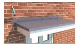
8.9 When the canopy is fully secured a second mastic sealant can be applied.
