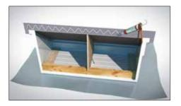
**5.1** Apply mastic sealant to the rear of the Flashing Upstand while on the ground. Use protective sheeting to front face of canopy.
