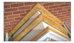
3.4 Secure the canopy through the timber frame at a minimum of 300mm centres using the recommended fixings and plugs (Fischer SXR 10x100mm).
