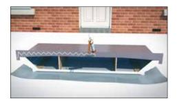
7.1 Apply mastic sealant to the rear of the Flashing Upstand while on the ground. Use protective sheeting to front face of canopy.
