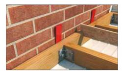
**8.4** Use packing shims to level canopy. Shims can be inserted from above or below as required.
