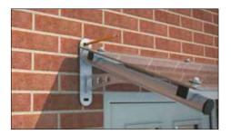
**4.2** To fit first bracket, mark positions for drill holes. Drill bit size M10.
