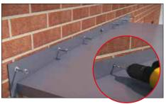
7.3 Secure the canopy by drilling through the flashing upstand at a minimum of 300mm centres with recommended fixings and plugs (Fischer SXR 10x60mm). Drill bit size M10.
