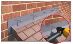
5.3 Secure the canopy by drilling through the flashing upstand at a minimum of 300mm centres with recommended fixings and plugs (Fischer SXR 10x60mm). Drill bit size M10.
