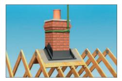
**4.1** Position the chimney ensuring it is aligned with the fixing support boards.
