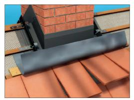
9.1 Ensure flashing is rolled back to clear working area. Secure extra batten to act as support for ply section. Note batten must extend further than flashing.
