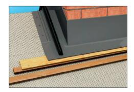
7.2 A batten and flashing support timber are now fixed in place under the bottom flange of the chimney. This provides support for lead flashing apron. It is important to ensure that this supports the lead sufficiently to prevent ponding.
