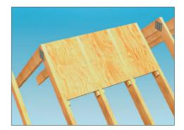
**1.3** Secure the fixing support boards between the rafters with stainless screws at 300mm centres into each batten.
