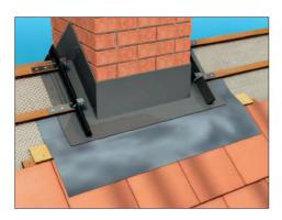
9.2 Fix ply section to tiling batten to create path for flashing to follow. When in situ, Dress the lead down over the tiles ensuring no ponding can occur.
