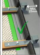
**8.3** Ensure batten fixings do not penetrate the secret gutter of the GRP fixing flange. When installing tiles including verge fixing clips, particular care must be taken to ensure a min 25mm gap remains between the tiles and GRP side cheek.
